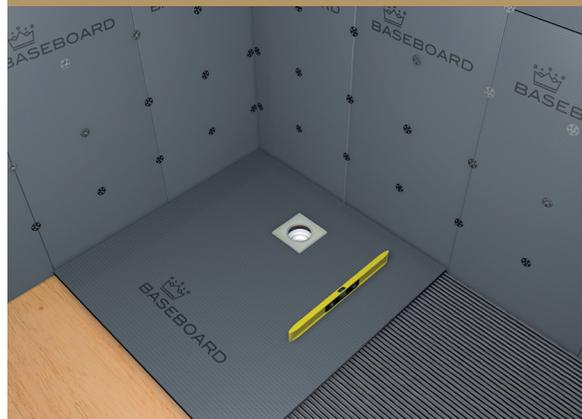
5. Insert the threaded collar to join the Baseboard Shower-Tray to the trap.
