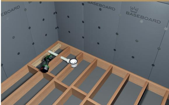
6. **Pro Tip** - The protection cap can be used to screw down the threaded collar by hand, and can be inserted to prevent dirt and debris entering the drain body until installation is complete.
