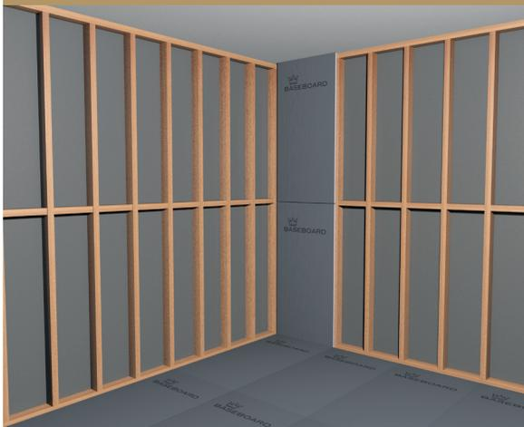
3. Fix using screws and washers at 300mm centres (vertical spacing) into each upright.
