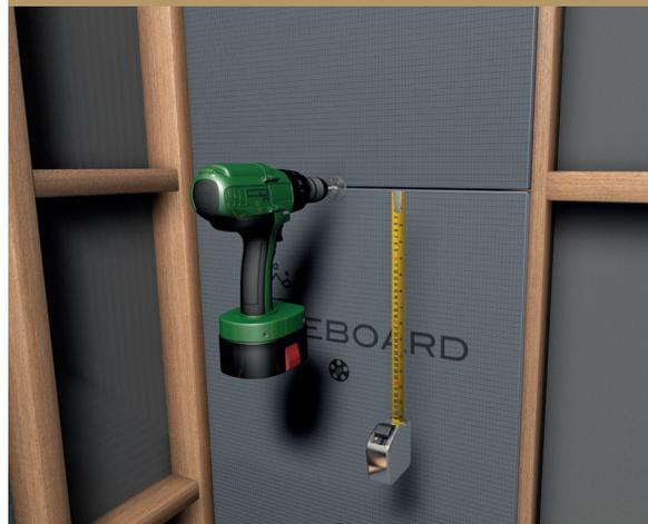
2. Ensure all board edges are supported with a vertical or noggin behind. Always make cuts before fixing.
