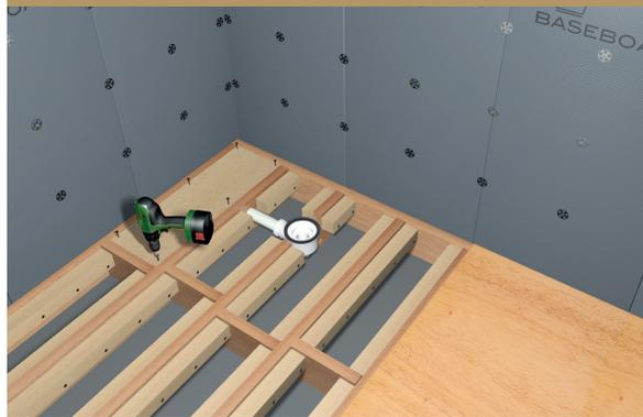
2. Solvent weld the trap into the waste pipe. **Pro Tip** – Check pipe is suitable for solvent weld and check connections are watertight before final installation of the Baseboard Shower-Tray.
