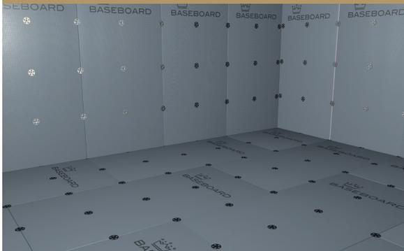
9. Once the adhesive is dry ensure to waterproof all joints with Baseboard Waterproof Tape (for wet zones - tape a minimum of 300mm past the wet zone area). Ensure all joints and screw heads are taped. If preferred, Baseboard AquaTank Fleece+ and Neo-Flex can be used for all board-to-board joints.
