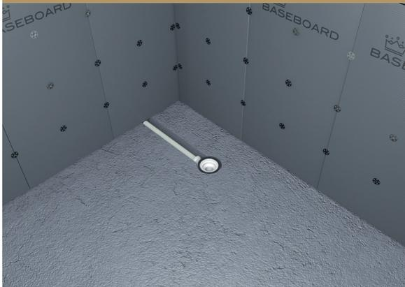
2. Ensuring the seal on the top of the trap is level with the surrounding subfloor, and the centre of the trap corresponds with the centre of the outlet in the tray, back fill around the waste pipe (using tile adhesive is ideal) and allow to set.
