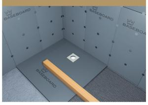
**4.** Check the installed Baseboard Shower-Tray is level on leading edges.
