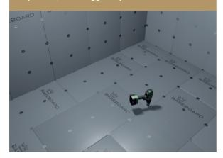
8. For this method, you can use offcuts to help create a brick-bond pattern - however, as a guide, do not use Baseboard offcuts smaller than 200x200mm.
