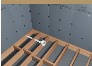
4. All plywood infill pieces must be fixed to the battens. Pro Tip – Mark the location of pipes and wires on joists before fixing plywood inlays.
