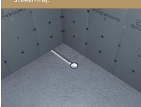
2. Ensuring the seal on the top of the tap is level with the surrounding subfloor, and the centre of the trap corresponds with the centre of the outlet in the tray, back fill around the waste pipe (using tile adhesive is ideal) and allow to set. Prime the floor using AquaTank Pro - Tile Primer before applying adhesive or Baseboard. Pro Tip - The correct notch size for combing out the adhesive bed is at least double the maximum undulation of the floor, measured under a 1m straight edge.
