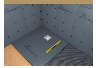
8. Once Baseboard Shower-Tray and remaining floor panels are in place, waterproof all joints with Baseboard Waterproof Tape (for wet zones - tape a minimum of 300mm past the wet zone area). Ensure all joints and screw heads are taped. If preferred, Baseboard AquaTank Fleece+ and Neo-Flex can be used for all board-to-board joints.
