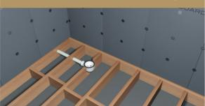
5. Carefully position the Baseboard Shower-Tray, ensuring alignment of the outlet in the tray with the trap. Apply a thin layer of adhesive and place the shower tray in position. Insert the threaded collar to join the Shower-Tray to the trap.
