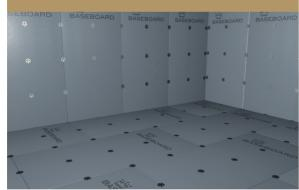
9. Once the adhesive is dry ensure to waterproof all joints with Baseboard Waterproof Tape (for wet zones - tape a minimum of 300mm past the wet zone area). Ensure all joints and screw heads are taped. If preferred, Baseboard AquaTank Fleece+ and Neo-Flex can be used for all board-to-board joints.
